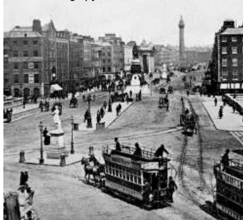
Photograph of O’Connell Street, Dublin, before the Easter Rising, by John L. Stoddard.
